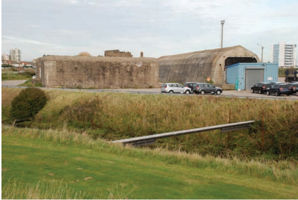
Figure 3. Stützpunkt 89 'Fulda' railroad gun bunker seen from D940 ©French Battlefields
